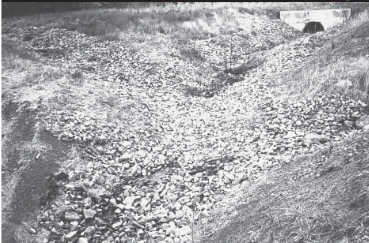
Plate 3.3 Rock Outlet Protection
